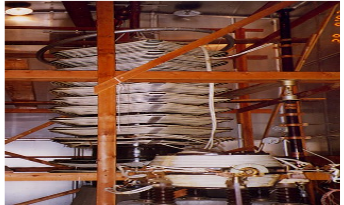
The old antenna tuning variometer, now retired. Moving it changes inductance to hold the antenna in tune.
