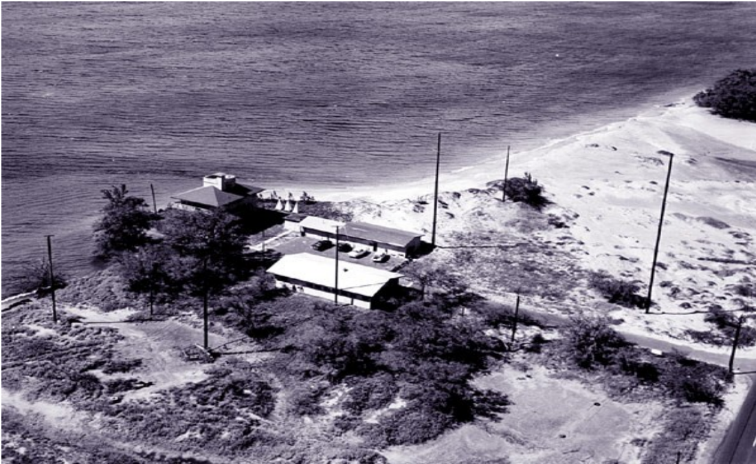
Kihei, Maui, 1948 to 1971. The original WWVH, right at the water's edge — the reason the station eventually had to move.
