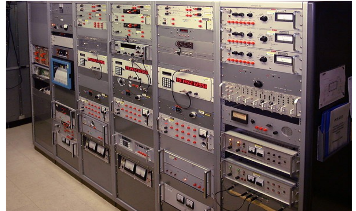
Kauai. WWVH's time and frequency rack: digital recorders, a multi-channel chart recorder, and the station clocks.
