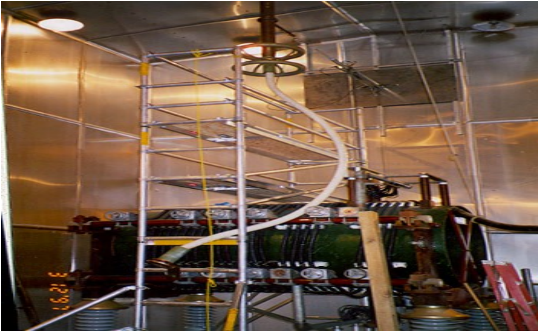
The helix house near completion. The white down lead is not yet connected to the antenna matching equipment.
