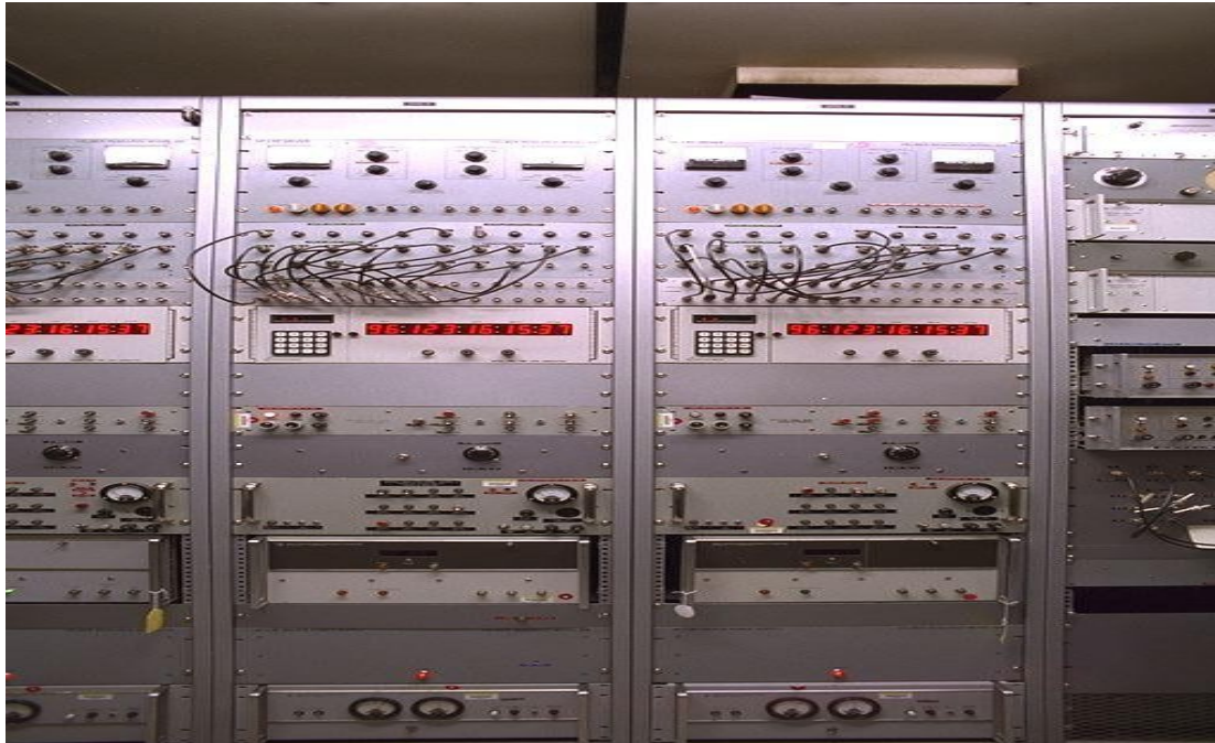
Fort Collins. The clock rack at WWV — the standards themselves, and the equipment that compares them.
